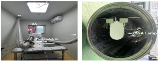
(a) Installation of heat exchanger (b) Photocatalytic reactor
