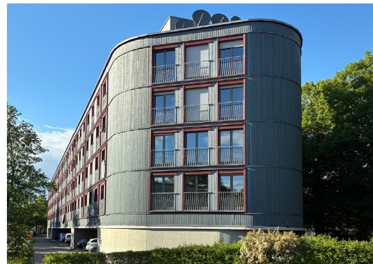
Fig. 8. South-facing facade, Wohnen am Dantebad, in 2026
