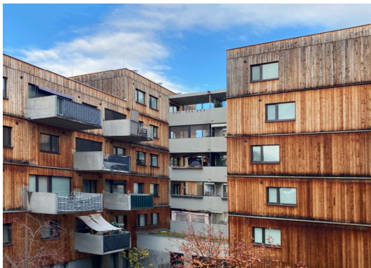
Fig. 5. Aspern D12 South-east facade, in 2024
