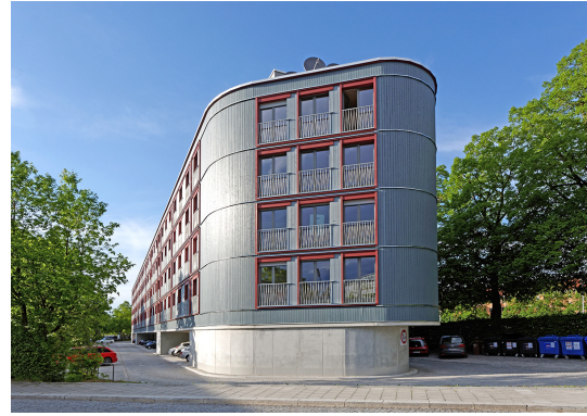
Fig. 7. South-facing facade, Wohnen am Dantebad, in 2018 (source: dataholz.eu)
