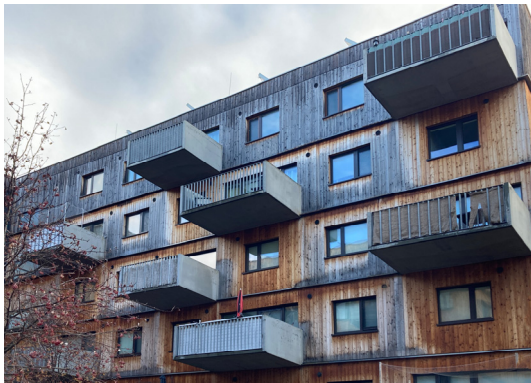
Fig. 6. Aspern D12 West-facing facade, in 2024
