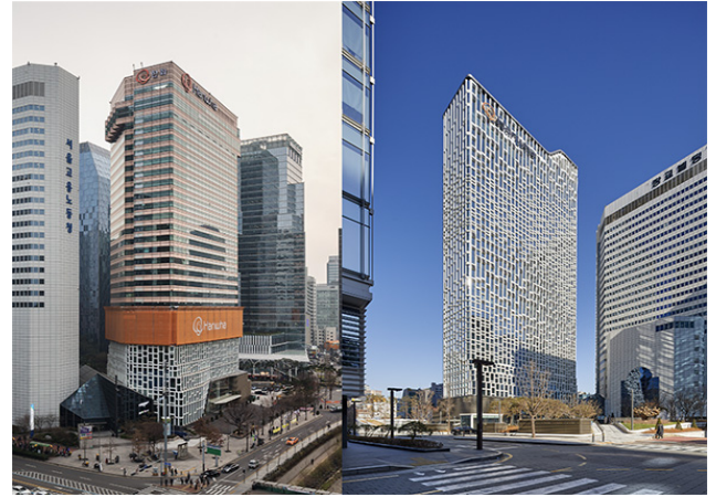
Fig. 2. Hamwha HQ During Facade Reconstruction (left) and After Completion (right) (photo: © Rohspace, courtesy of UNStudio)
