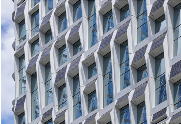
Fig. 5. BIPV Integrated Facade (photo: © Rohspace, courtesy of UNStudio)
