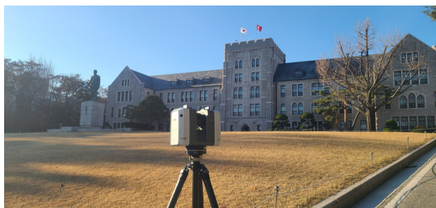
Fig. 1. 3D scanning of Korea University Main Building
