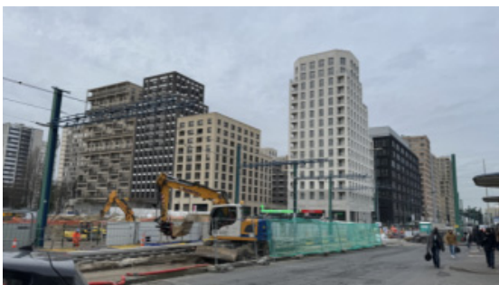
Fig. 13. View from the bus station (2025)
