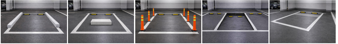
Fig. 3. Parking block line Fig. 4. Center block Fig. 5. Flexible bollard Fig. 6. Parking trench Fig. 7. Rumble strips
