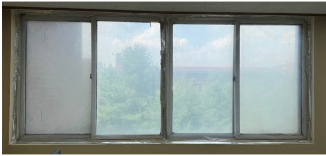
a) Architectural components
