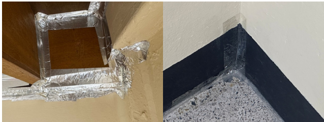
c) Miscellaneous envelope leakage components
