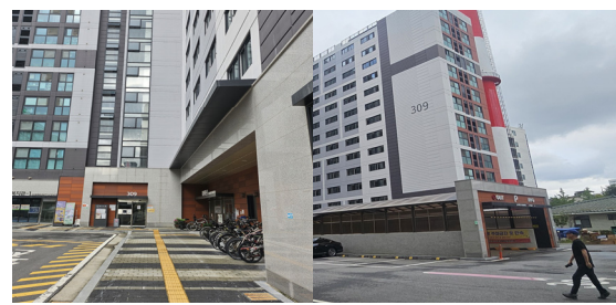
a) Pedestrian entrance b) Vehicle entrance
