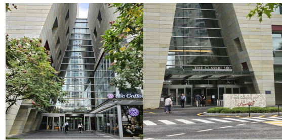
a) Pedestrian entrance b) Vehicle entrance
