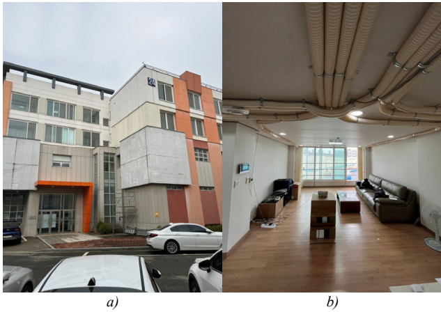
Fig. 1. Test building and living room
