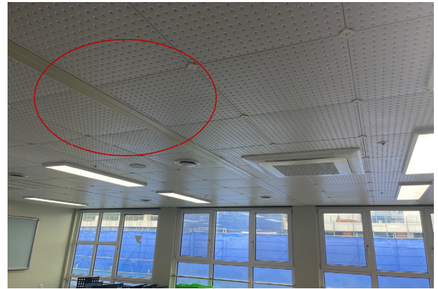
Fig. 9. Ceiling materials of B elementary school
