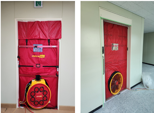
Fig. 3. The Installation of The Bower Door Equipment
