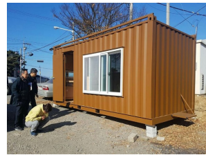
Fig. 3. Picture of Pohang temporary housing 1
