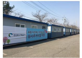
Fig. 4. Picture of Pohang temporary housing 2
