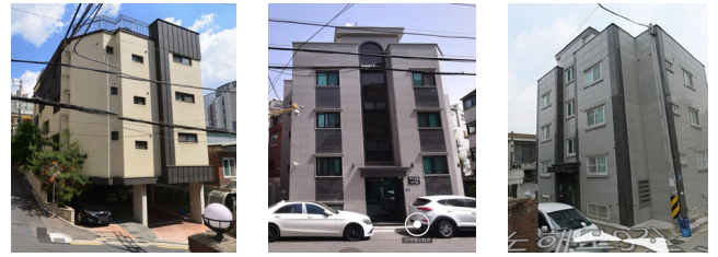
Fig. 6. Window shapes and arrangements; case A, D & H (images from Naver street view)
