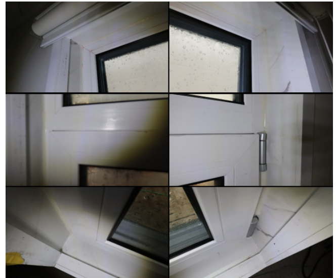
Fig. 11. Checking for window waterproofing performance
