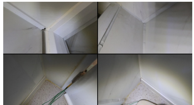
Fig. 12. Checking for corner and angle waterproofing performance
