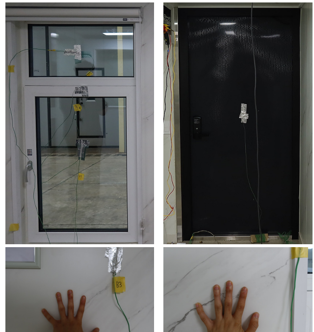
Fig. 9. Checking for condensation in a modular house (Order of windows, doors, and walls)
