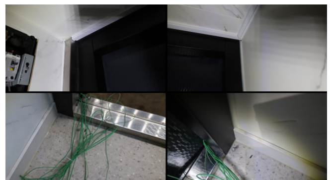
Fig. 13. Checking for door waterproofing performance
