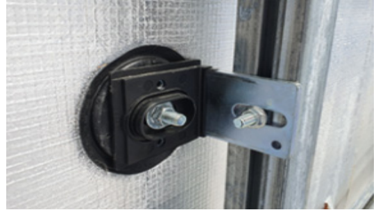
Fig. 3. Examples of thermal breaking anchors
