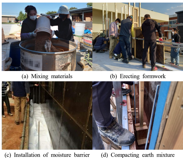
Fig. 2. Execution procedure of in-situ rammed earth wall
