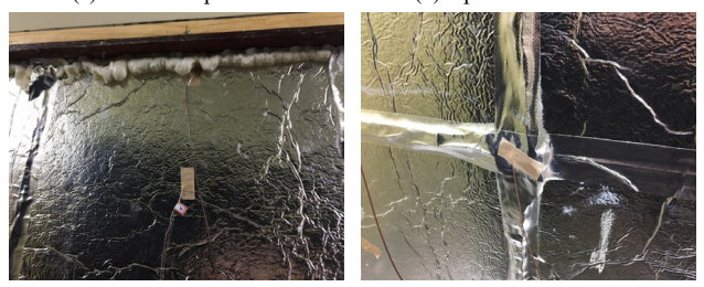
Fig. 9. Installation of VIPs applied walls
