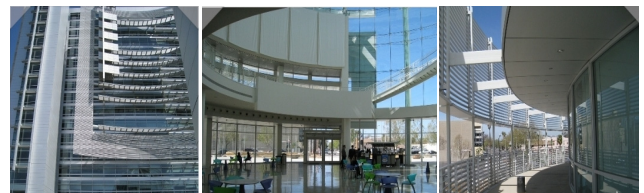
Fig. 20. Exterior and interior views of San Jose City Hall
