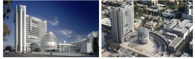
Fig. 18. Photos of San Jose City Hall
