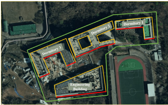
Fig. 5. Location of case study buildings(G campus)
