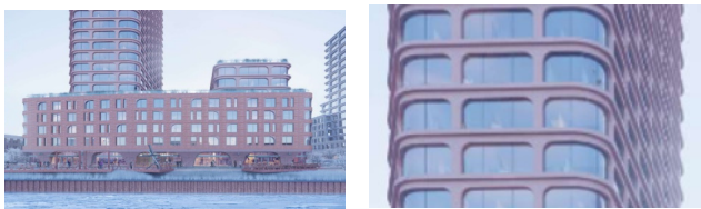
Fig. 12. Over-sized arch in 300 Nevins podium, and tower façade, designed by Fogarty Finger Architecture.
