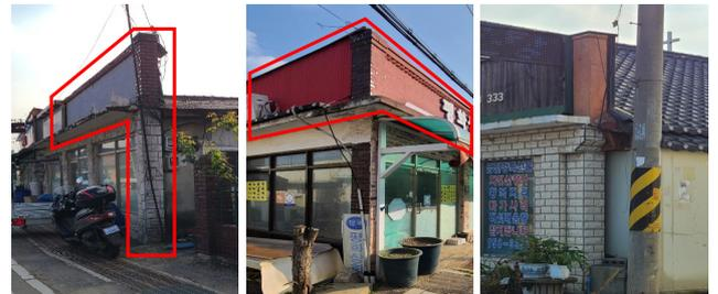
Fig. 14. Front integrated exterior wall type and roof slab railing wall type
