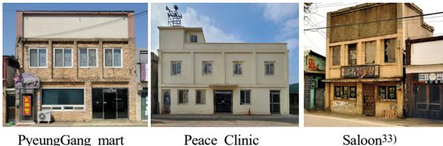
Fig. 25. Emphasizing the facade with columns and slabs standing out
