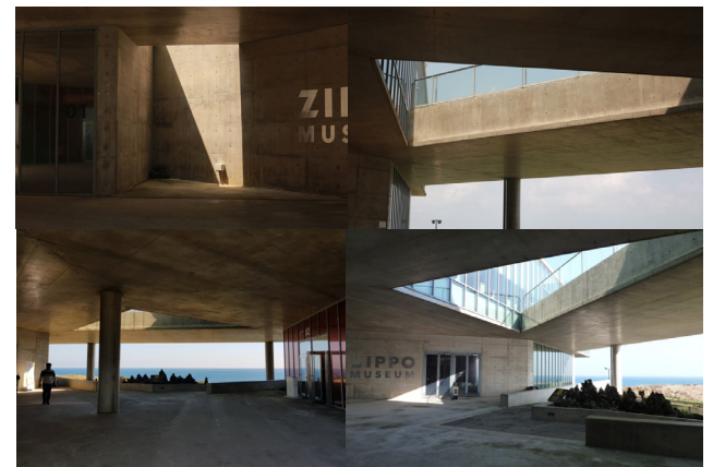
Fig. 26. Triangular opening for natural light on the deck
