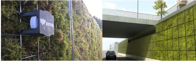
Fig. 3. Moss Module Panel (Source: www.achilles.be/case/besix-group/)
