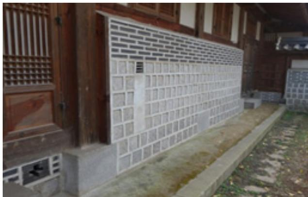
Fig. 10. The chimney on the wall of the Boksudang
