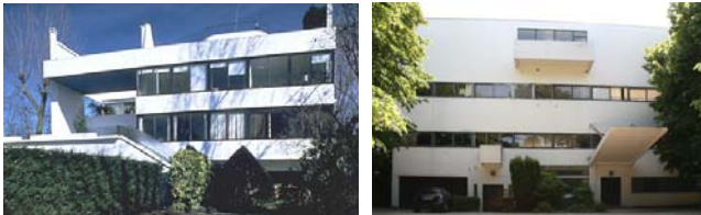
Fig. 23. Exterior View of Villa Stein
