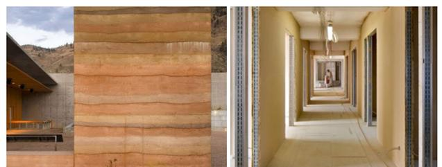
Fig. 5. Rammed earth Fig. 6. Earth panel
