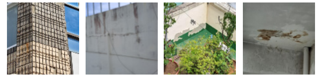
Fig. 3. Part of defect occurrences about the leak
