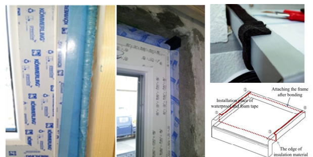
Fig. 5. Details of the construction for the window
