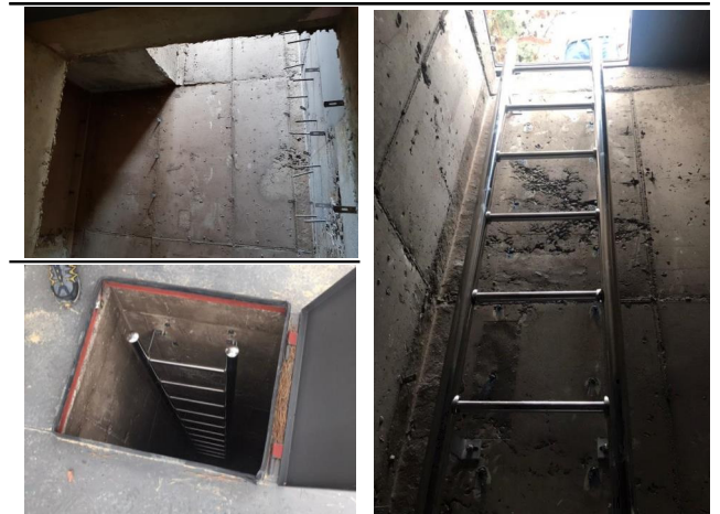
Fig. 3. Emergency Exit and Filter Room Construction of Shelter
