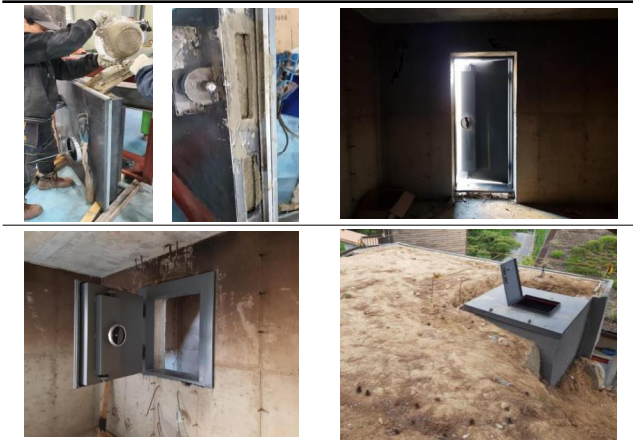
Fig. 4. Blast door Construction of Shelter
