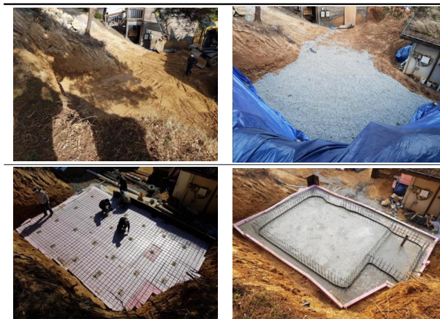
Fig. 1. Foundation Construction of Shelter
