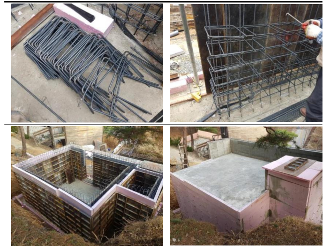
Fig. 2. Framework Construction of Small Scale shelter
