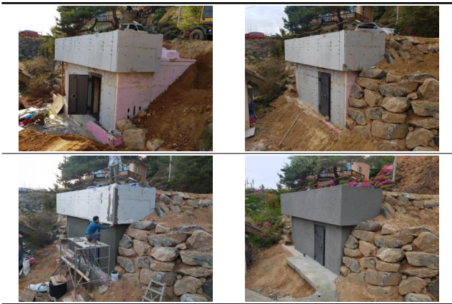
Fig. 5. Finish Work and Back Filling of Small Scale Shelter
