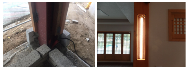
Fig. 7. H-shaped Steel + Wood Junctional Structure - Eunpyeong Community Center
