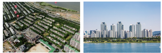
Before : Sinbanpo 1 Apt After : Acro River Park Fig. 8. Before and After Reconstruction (Sources : [5])
