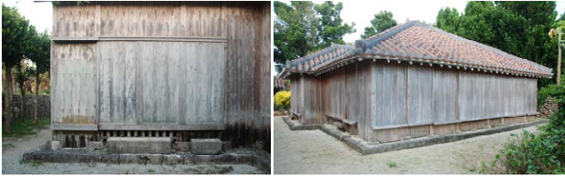
Fig. 19. Detail of sliding shutter door(Amado, あまど)
