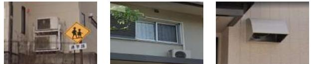
Fig. 16. Location of Outdoor condenser location & Exposed piping cover & Ventilation cap Shape
