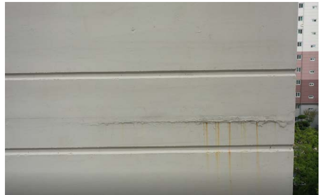
Fig. 4. Defects of exterior wall
