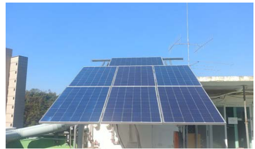
Fig. 1. The PV system being monitored
