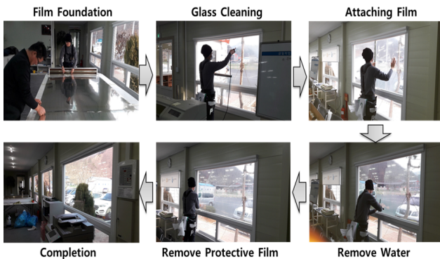
Fig. 8. Construction Process of Low-e Film
