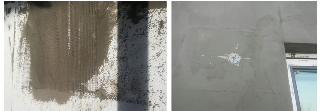
Fig. 1. Mesh (Left) and Fasner (Right) Used When Installing Dry-bit
