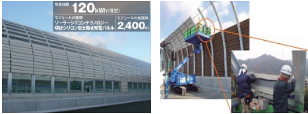
Fig. 5. Japan PV soundproof wall Installation Cases
