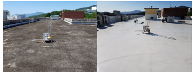
Fig. 7. Measurement of rooftop characteristics(NCR-left, CR-right)
