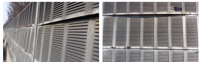
Fig. 1. Deteriorated noise barrier
