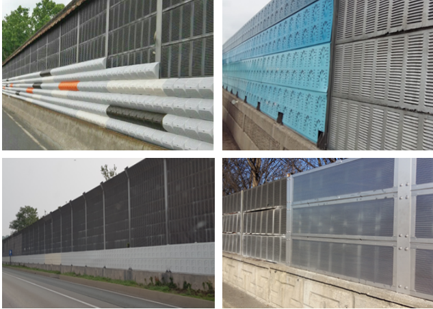
Fig. 2. Remodeling of deteriorated noise barrier
