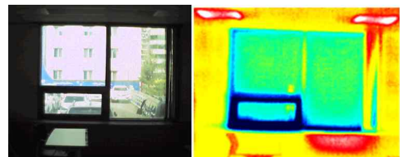
Fig. 6. A thermographic camera image of an existing window
