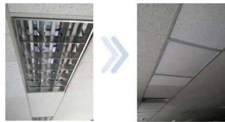
Fig. 3. Replacement of lighting fixtures
