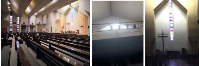
a. Daylighting of Interior Area b. Toplight of Altar c. Sidelight of Altar Fig. 36. Daylighting in Bulgwangdong Cathedral
