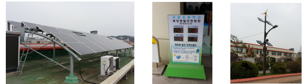
Solar Facility Solar status board Solar Lighting Fig. 9. Energy-efficient elements of Jecheon uirim Elementary School
