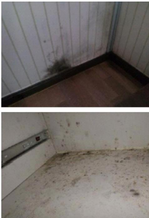
Fig 1. Examples of condensation in walk-in closet
