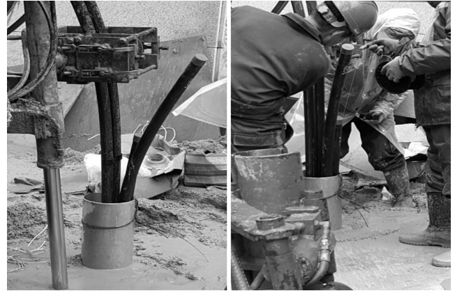
Fig. 4 Double U-tube and thermo couple installation
