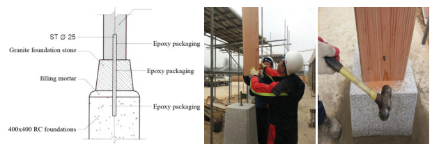
Fig. 2. Details of join the Foundation column
