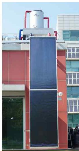
Fig. 4. Natural circulation solar hot water system installation
