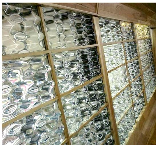
Fig. 1. Water-filled trombe wall concept (An idea of Solar Decathlon team from University of Arizona in 2009)
