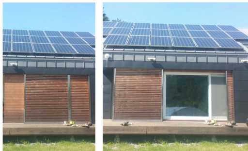
(a) closed louver Fig. 7. Moveable louver
