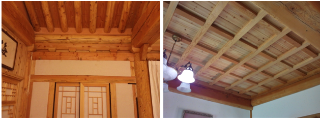
Figure 4. Exposure or not of Wooden members(lining room)
