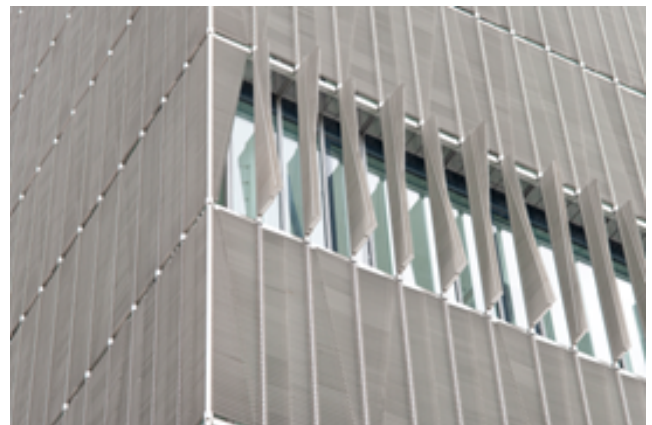
Fig. 2. ThyssenKrupp Quartier https://www.thyssenkrupp.com/en/presse/bilder.html&photo_id=1126 (accessed on 16 January 2016)
