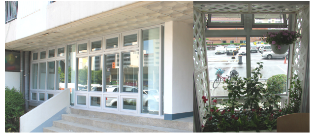
Fig 4. Status on Double windows installation and plant layout
